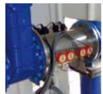
**DOMESTIC SUPPLIES** | **atg UV Technology** have provided UV disinfection systems for the treatment of potable drinking water for individual properties and small village supplies around the world, typically treating between 2 and 14 m<sup>3</sup>/hr in a single high output low footprint system.
